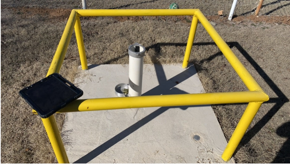
Figure 9: Well 221266 installed at Sharon Oklahoma, 06/07/2023.
