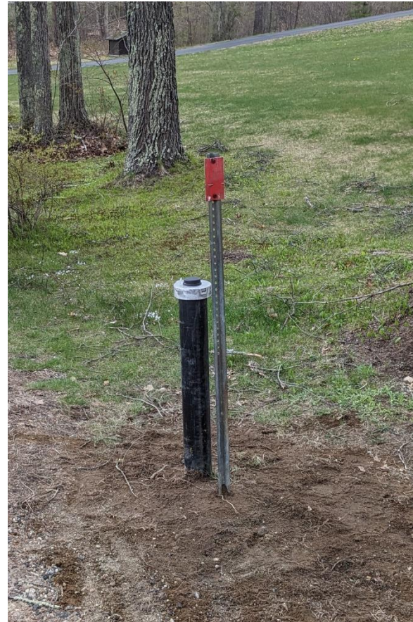
Figure 1. Photos of the protective surface casing of BBW-53 before (left) and after (right) replacement of the surface protective casing.
