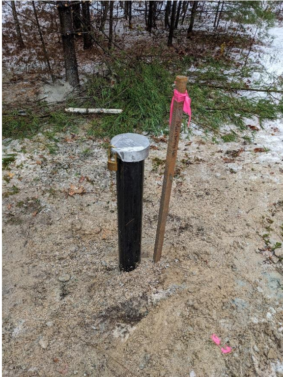
Figure 2. Protective surface casings for replacement overburden well LMW-36 (left) in Litchfield, NH and NGWMN expansion well KEWB-01 (right) in Keene, NH,
