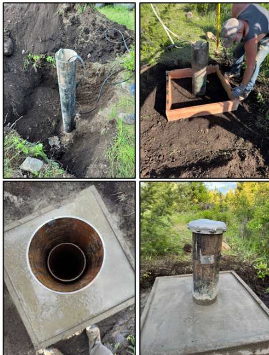
Figure 15. MBMG-6024 well rehabilitation.
