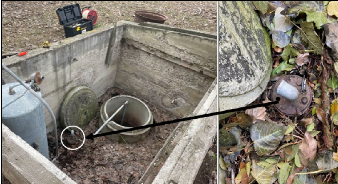
Figure 5. MBMG-133880. The well is located in the foundation of an old building. Pump and drop pipe are still in the well and could not be removed. Lack of cell coverage prevented successful GPS survey. Location updated with navigational GPS.
