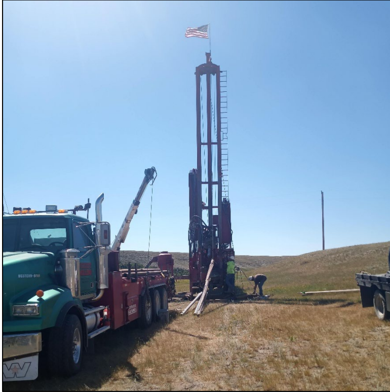
Figure 9. Wells were drilled using a dual rotary rig.
