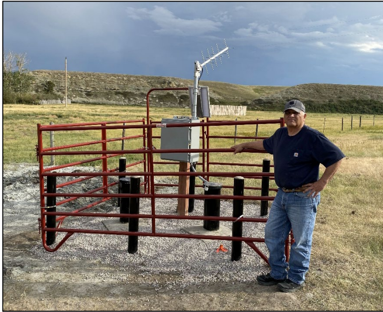
Figure 11. Completed well pair.
