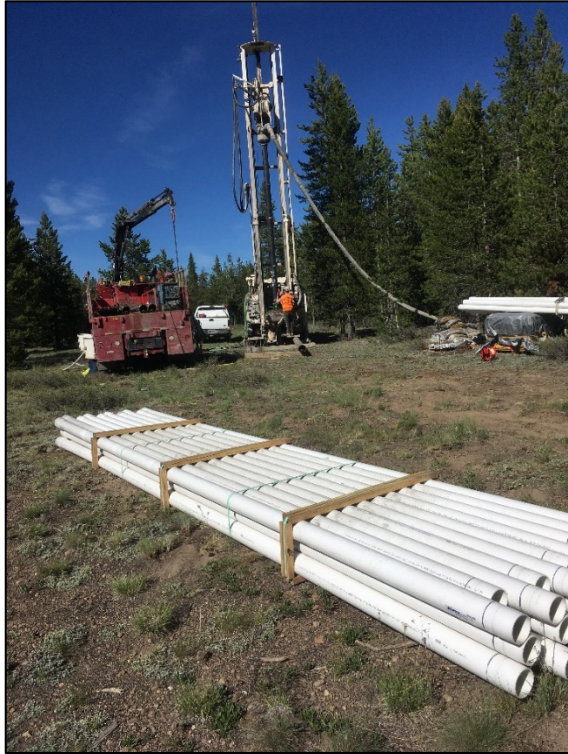
Figure 2. The wells were drilled using a dual air rotary drilling rig.
