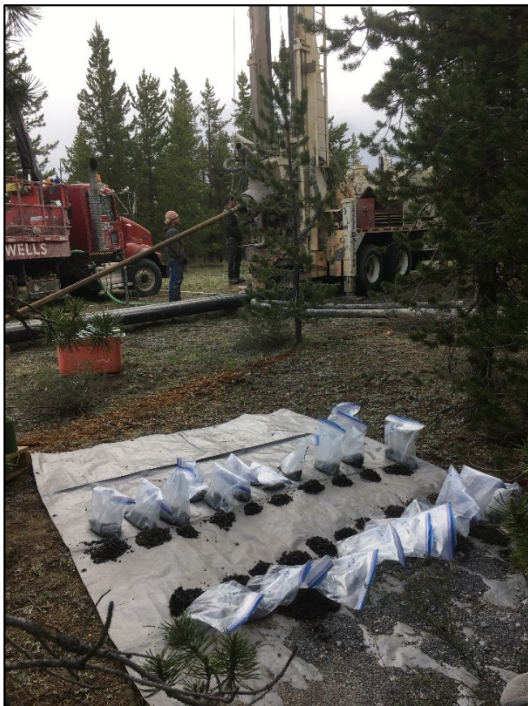
Figure 3. Cuttings were logged onsite.
