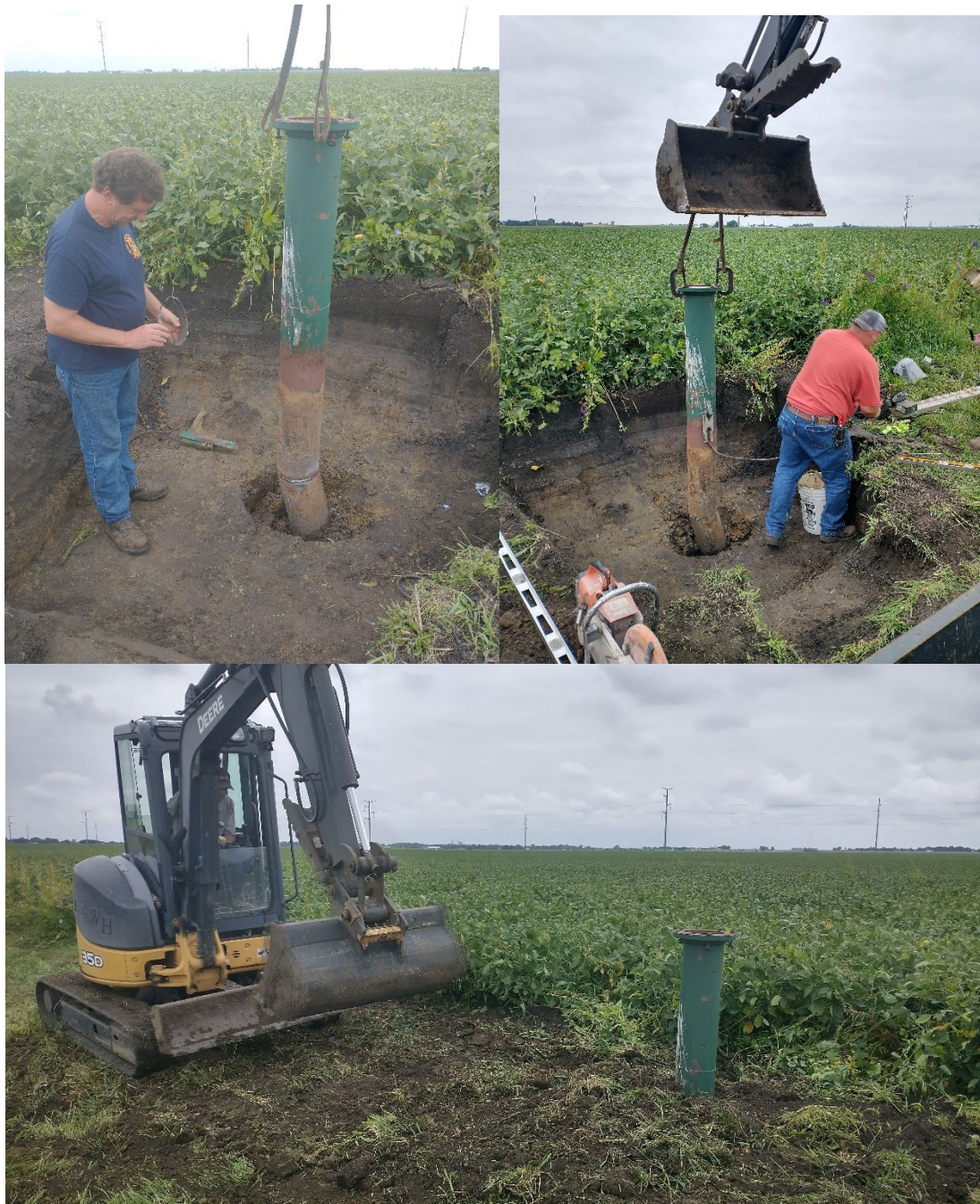
Figure 4. Photographs of the Petro North NGWMN well being repaired in September 2023.
