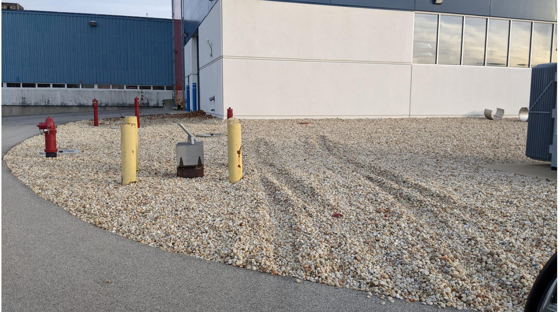
FIGURE A3. FERMILAB WELL #2 (API 120430206300) AT SITE 1 SURROUNDED BY PROTECTIVE BOLLARDS.
