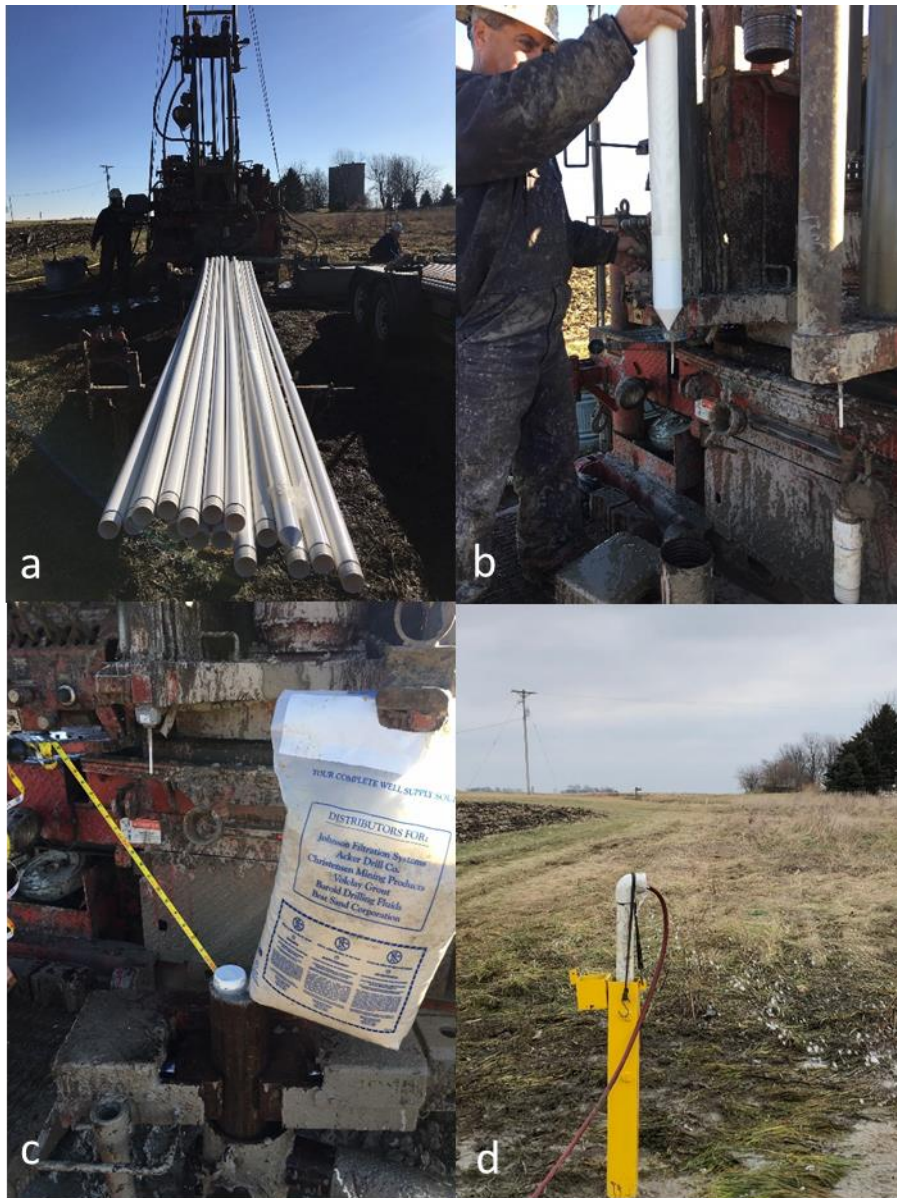
Figure 8. (a) 2-inch PVC casing and screen ready for installation, (b) installing well screen, (c) installing sand pack (d) completed wellhead protector during air-spurge well-development. All photos are from the KENN-20-02 site at Rowell, Illinois.
