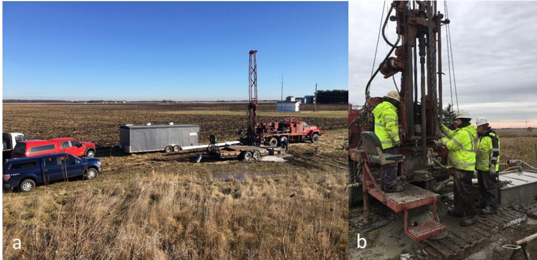
Figure 2. (a) Perspective view of CME drilling rig system operated by the ISGS and (b) extraction of continuous core from the wireline sampler. Photos are from the KENN-20-02 site at Rowell, Illinois.
