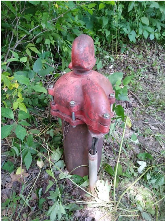
Figure 18. Starved Rock after cleaning and installation of new bolts
