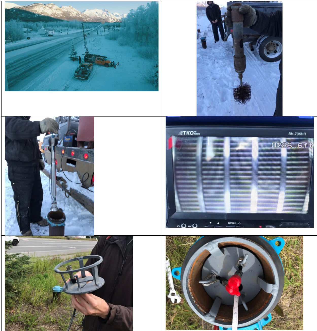
Fig. 5 Eagle River, Alaska - Monitoring Well Rehabilitation (USGS grant #G16AC0036) conducted in February 2020, Well ER-5 confined, mid-valley aquifer, previously monitored by Alaska Department of Geological and Geophysical Survey (DGGS) from 1983–1991. Upper left: M-W Drilling boom on Eagle River Rd; upper right: sweep/brush unit used to clean well screen, middle left: pump used to purge well; middle right: cleaned well screen at 296 ft depth; bottom left: custom fabricated well hanger plate; bottom right: ER-5 well logger installation with pressure transducer and barometer anchored in well hanger plate set in well casing.
