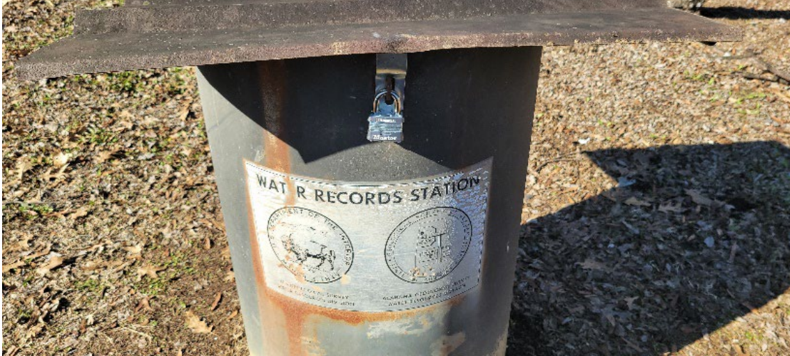
Figure 4. Trend well GSAL 125301 (JAC-2) after repairs. Photo illustrates cover secured by new hasp and lock.
